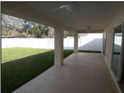
Huge covered lanai with ceiling fans, and large fenced back yard.
